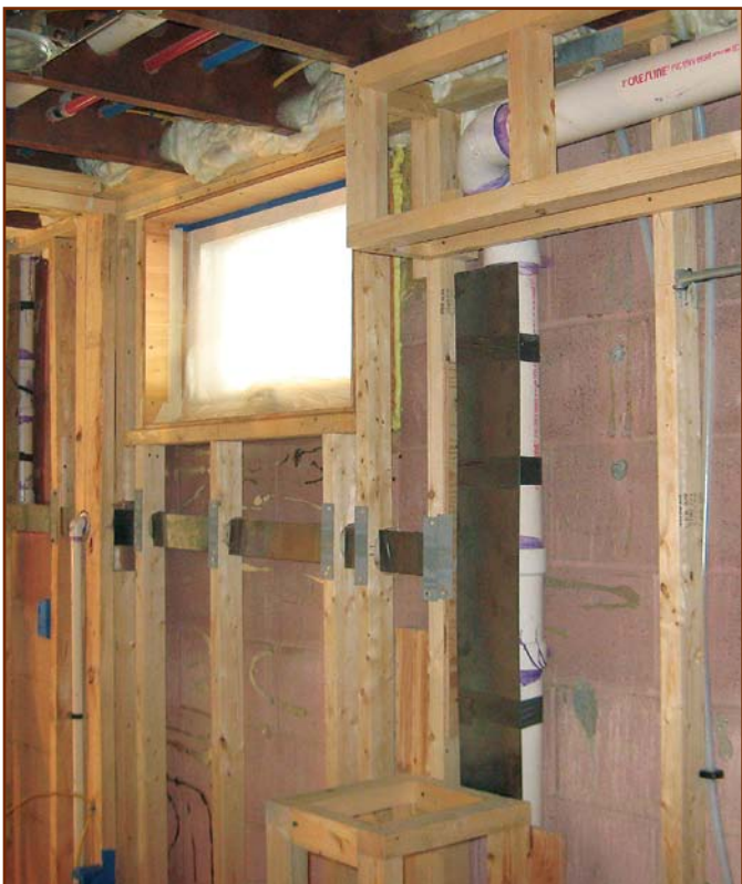
A better basement wall. The basement of the 1960s ranch was typical of the era—damp, cold, and uncomfortable. To insulate the original block foundation, we framed new 2x3 stud walls 2 in. away from the original block wall. Filling the resulting 4½-in.-deep cavity with closed-cell spray foam yielded an improved foundation assembly of R-27.
