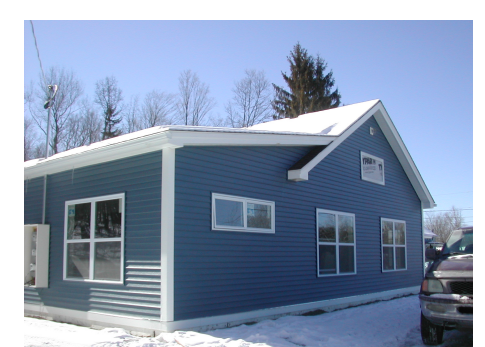
Reconstruction of a Commercial Building Route 44/55 - Marlborough / Highland ICF frost wall, spray foam insulation in walls and rafters, radiant heat, heat recovery ventilator Extremely efficient to heat and cool
