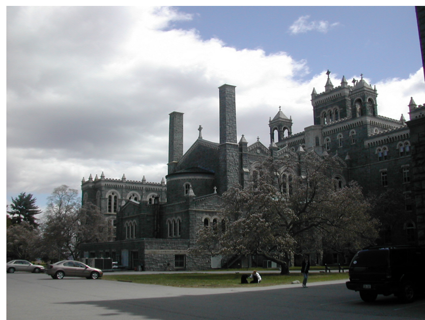
Mount St. Alphonsus in Esopus on the Hudson River 150,000 +/- sf - c. 1908 with a spectacular chapel Precise as-built floor plans (completed in 4 weeks) Code compliance review for existing conditions and renovations
